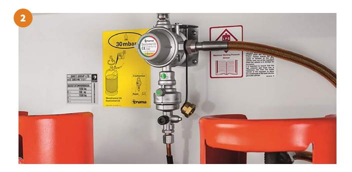
Check the age and condition of the high pressure gas hose and regulator, and replace if required.
