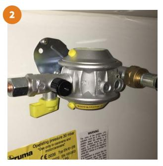
Open the safety drain valve (yellow handle) next to water heater, and leave open.
