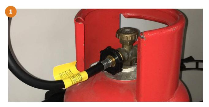
Ensure the gas supply is isolated at the gas bottle, and ensure that the gas manifold taps are off.
