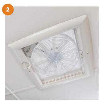
Ensure all fixed ventilation points (high and low) are clear from debris and obstructions.
