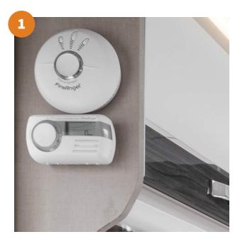
Check the battery expiry date on the smoke alarm and replace or remove as required.
