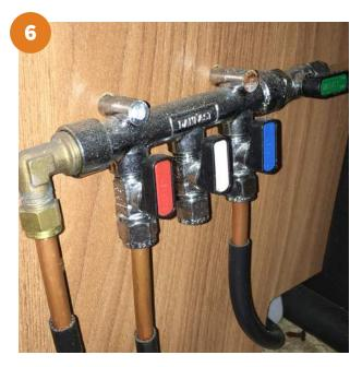
Disconnect the inlet pipe to the onboard water pump, mesh filter and outlet pipe, and re-run the pump for a short time, to ensure all the water is removed. Leave the system disconnected during storage.
