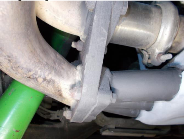
Fixing bolts good
